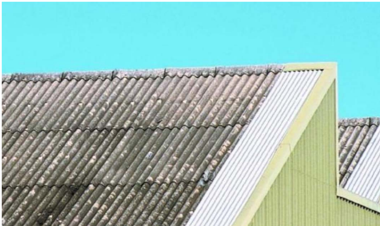
Factory Roof, Photo – SafeWork SA
